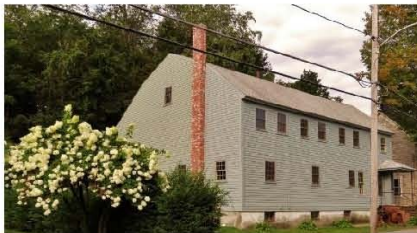
How the Grange Hall looks today after new siding, new windows, and a new chimney.
