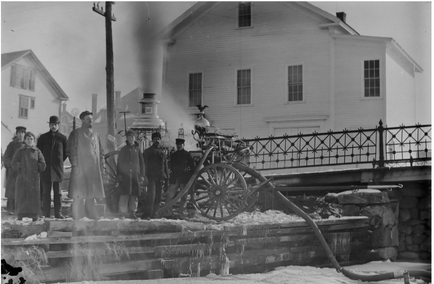
Baldwinville in the late 1800's testing out the steamer in front of the old Tiger #1 fire station. The Narragansett Hotel is the building on the left.
